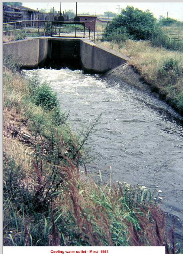
Cooling water outlet - Most 1968
